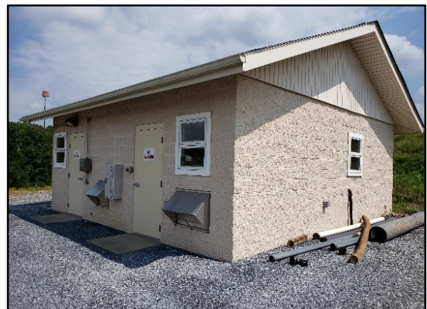
GLRA Leachate Pump Station No. 7
