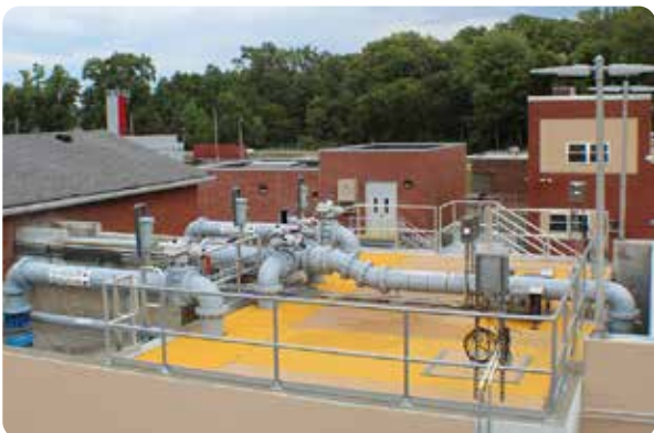
An AquaStorm ® system operating at a municipality for dual tertiary/wet weather treatment.
