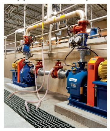
In many industrial applications, including poultry processing plants and pulp and paper mills, Super T Series® pumps equipped with the Eradicator® Solids Management System keep feathers, rags, bags and debris from coagulating around the eye of the pump's impeller.
