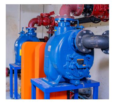
The removable inspection cover of these RAS and WAS pumps in a small WWTP makes it easy to remove an obstruction should one occur.
