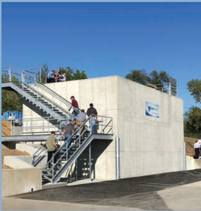
AquaNereda® Demonstration Plant
