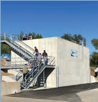
AquaNereda® Demonstration Plant
