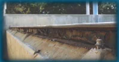
Corroded Rails
