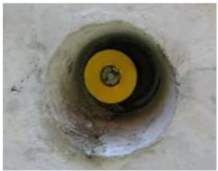
Anchor pocket with single strand tendon & wedge set
